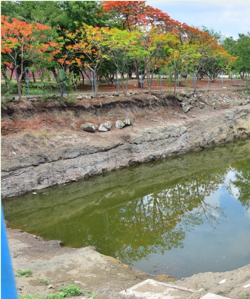
Rain water harvesting panoramic view of water tank 10 million Litres capacity.
