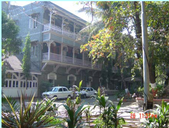
CRIME BRANCH BUILDING, MUMBAI
