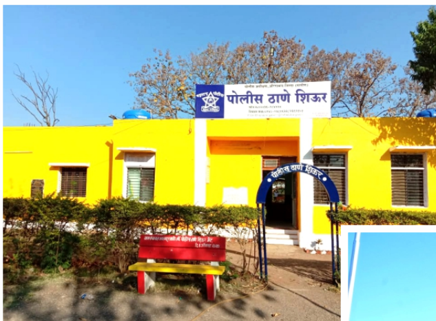
Shiur Police Station
