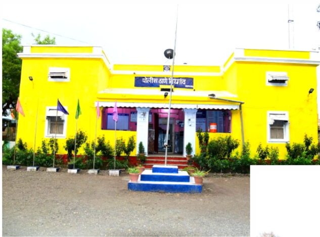
Virgaon Police Station
